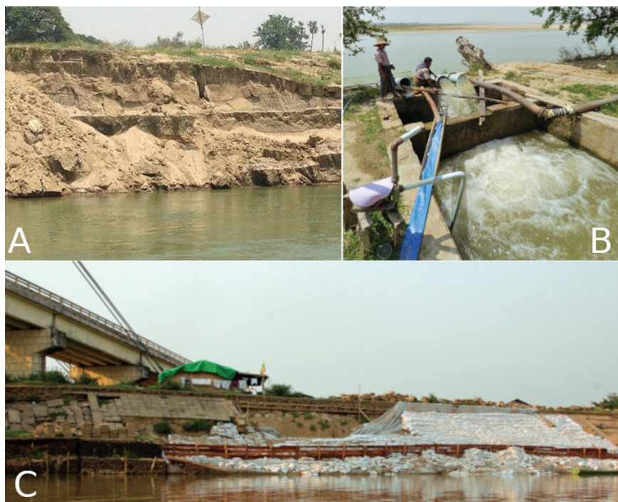
Figure 5.1 A. Bank erosion along the Chindwin River (photo: Chayanis Krittasudthacheewa, Apr. 2014); B. Pumping station of irrigation canal where farmers reported risk of bank erosion, Chindwin River, downstream from Monywa. (photo: Chusit Apirumanekul, May 2015); C. Sandbags and cement plates being placed to protect bridge from bank erosion, Homalin (photo: Vitor Vasconcelos, May 2015).
