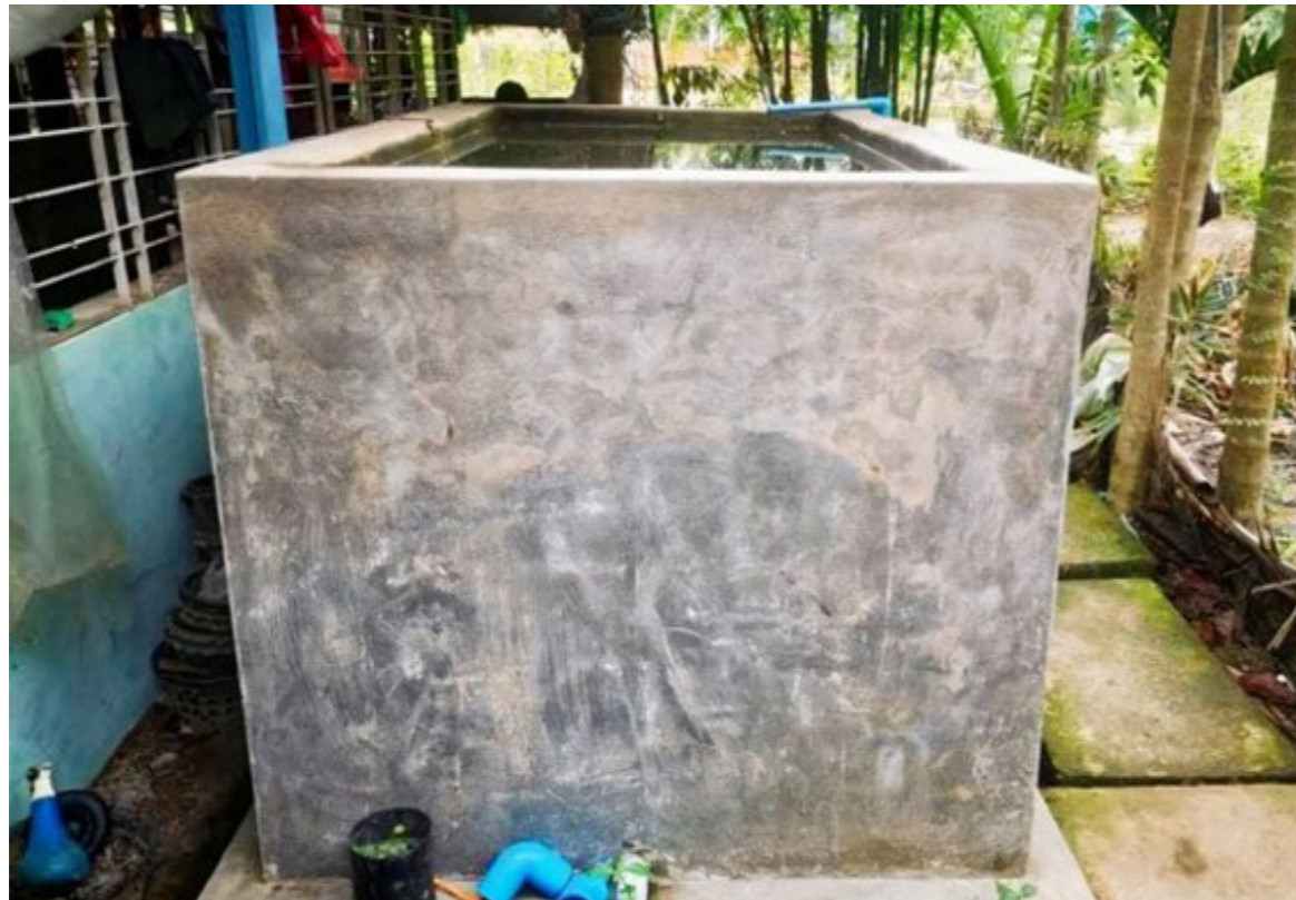
Concrete storage tank in Bogalay suburban area. Photo by Dr. Nilar Aung
