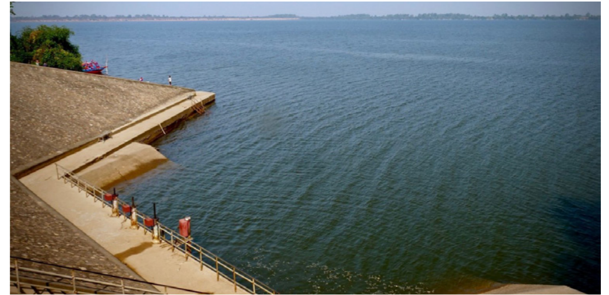
The Angkor-era reservoir holds 56 million cubic metres (1.98 billion feet) of water and supplies Siem Reap city with 17,000 cubic metres (600,349 cubic feet) of water per day which accounts for more than half the city's current daily capacity, according to the Siem Reap Water Supply Authority. The West Baray also supplies more than 10,000 hectares of farmland with irrigation but there is not enough to meet farmer demand in the dry season, according to APSARA, which manages the reservoir. Photo: Jack Brook for Southeast Asia Globe
