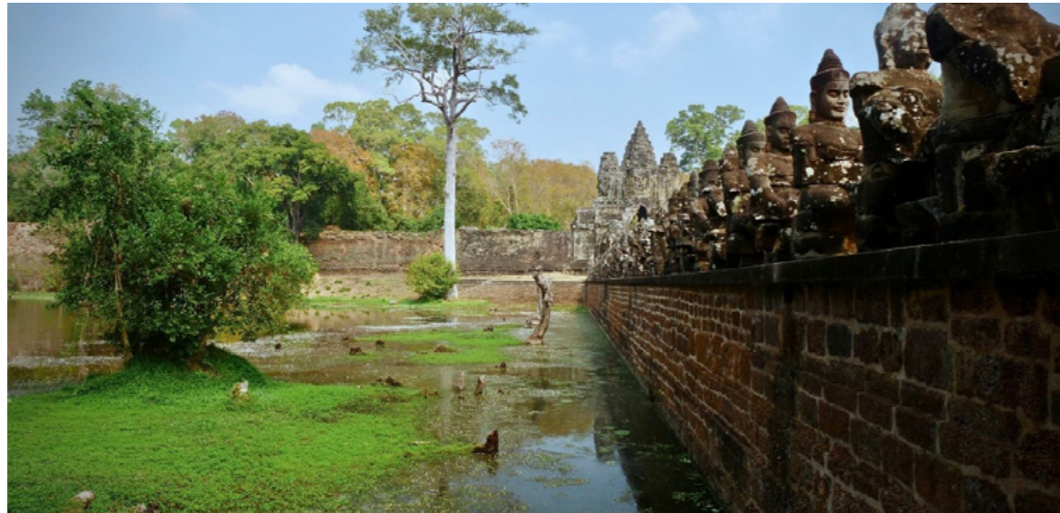
The moats, reservoirs and canals within the Angkor Archaeological Park are overseen by APSARA and, alongside underground water tables, are important for stabilising the bigger temples.
